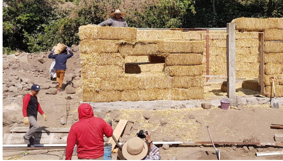
(The picture shows one of the amazing “hay bale” houses under construction, that some of our coworkers in Puebla have helped with, and some of you have helped fund.)
